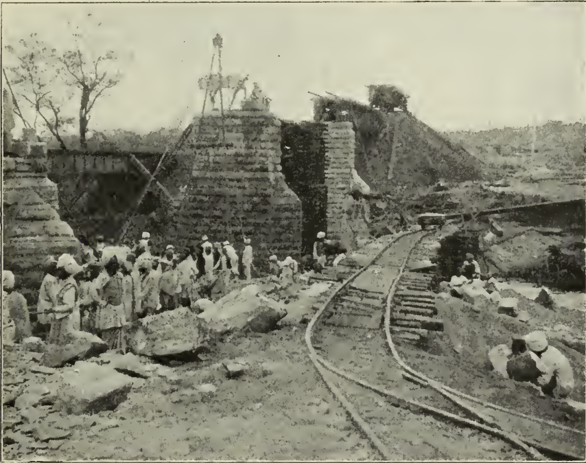
“THE HEAVY STONES WERE SWUNG INTO POSITION.”
